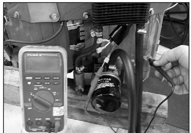
Figure 7-2. Testing DC Output Wire
