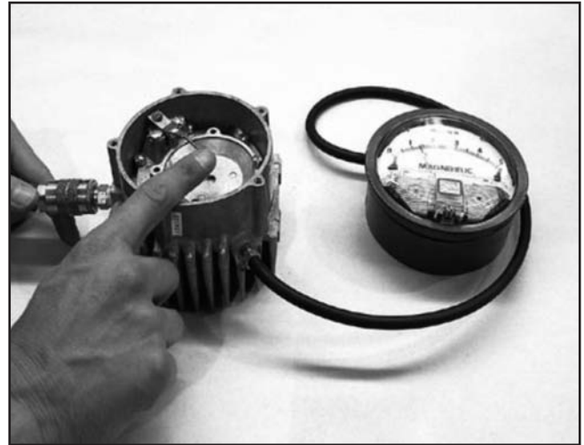
Figure 3-26. Check Primary Pressure Reading
